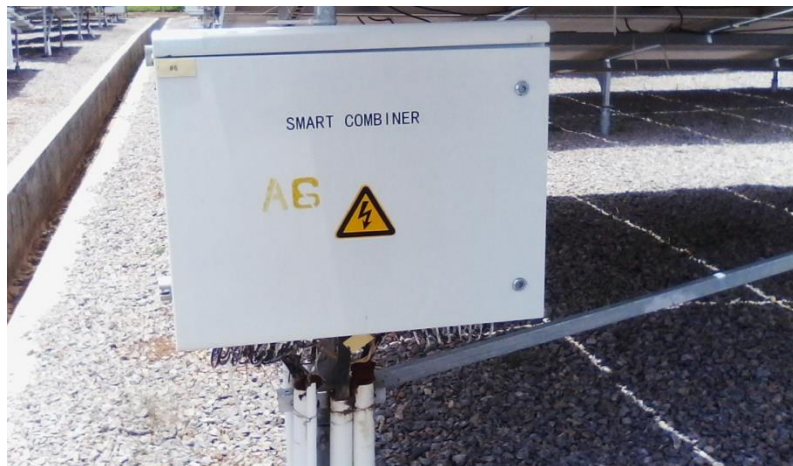
Figure 3.3 Array Combiner Box at Navrongo VRA Solar Plant
