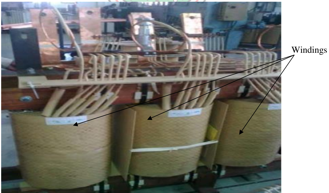
Figure 2.7 Three Phase Transformer Windings
