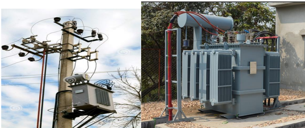
Figure 2.4 Pole Mounted and Ground Mounted Distribution Transformers
