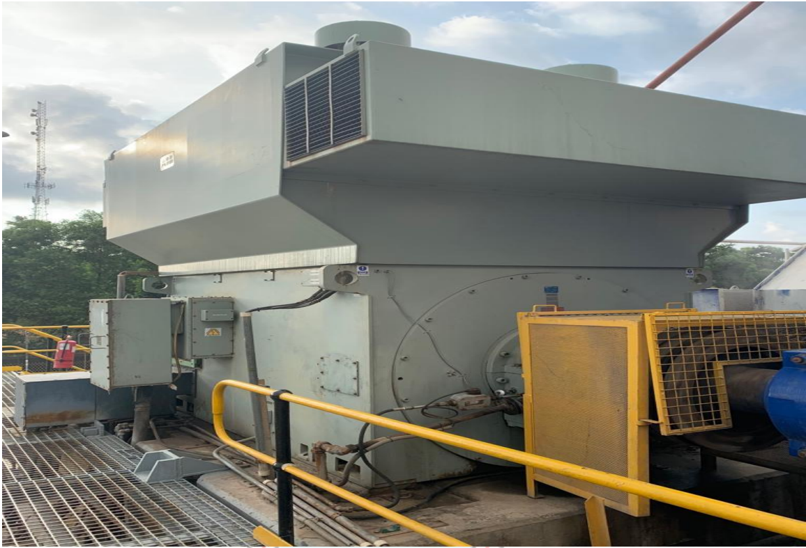
Fig. 3.2 Drive Side of the SAG Mill Motor
