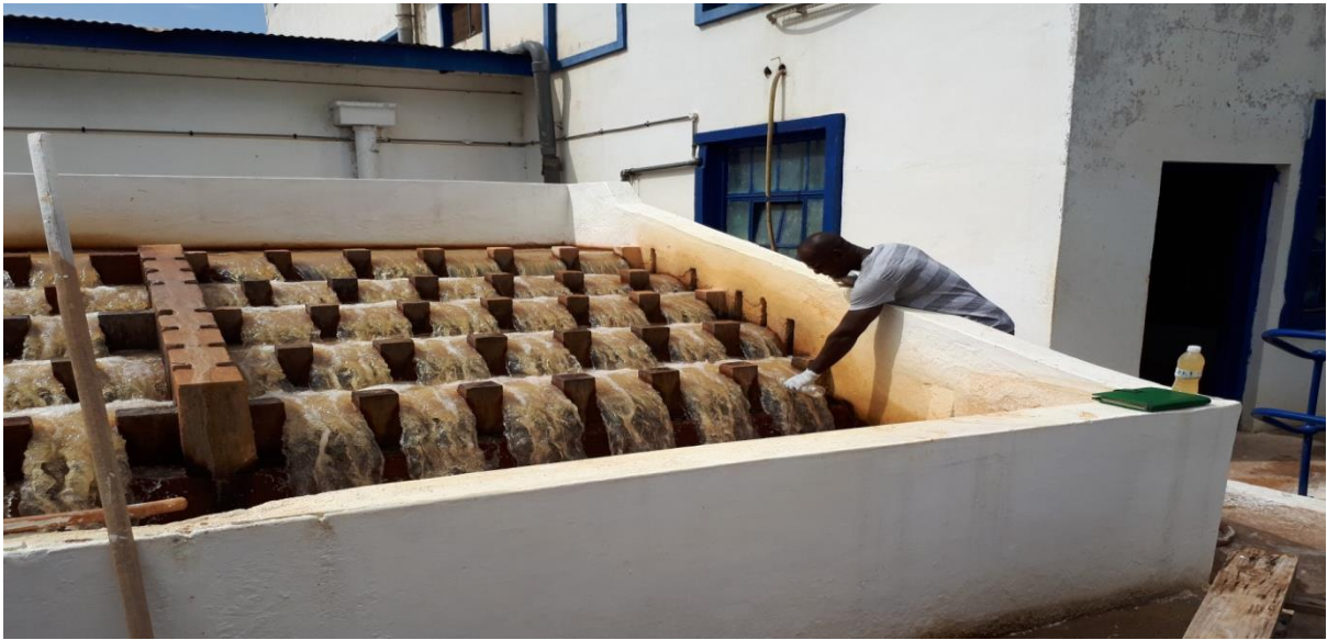
Figure 2.11 OWTP Cascade Aerator
