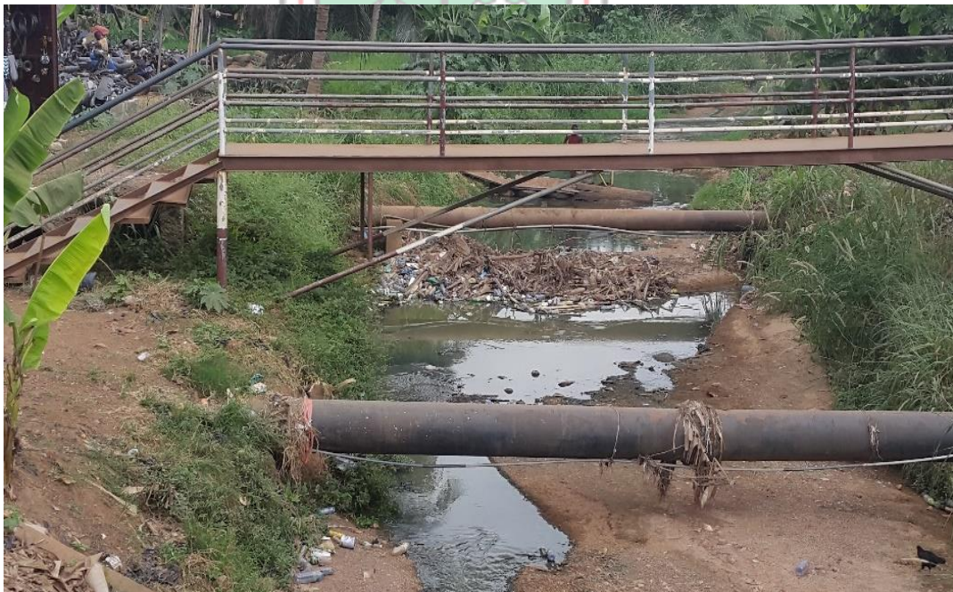
Figure 5.2 18-inch and 14-inch mains from Owabi to SWR passing through drainage carrying effluents from the Abrepo community
