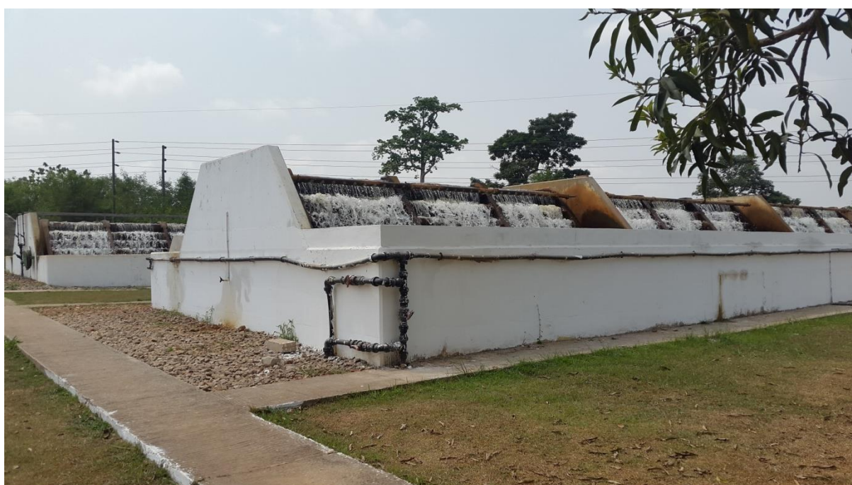
Figure 2.5 Double Cascade Aerator at BWTP
