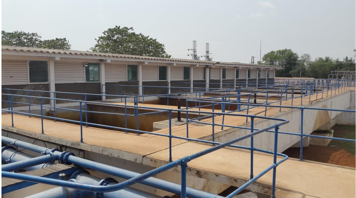
Figure 2.8 BWTP Sand Filters
