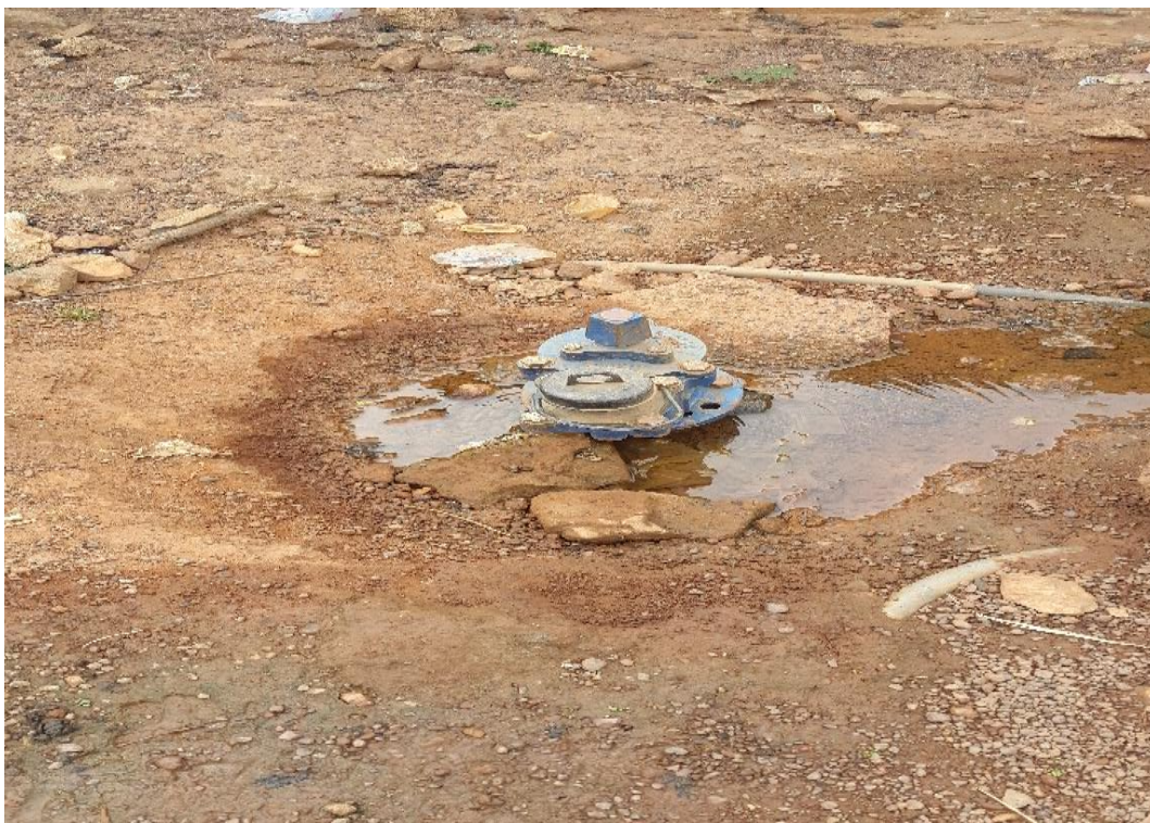
Figure 5.3 A leaking dead-end blow-out at Nkawie
