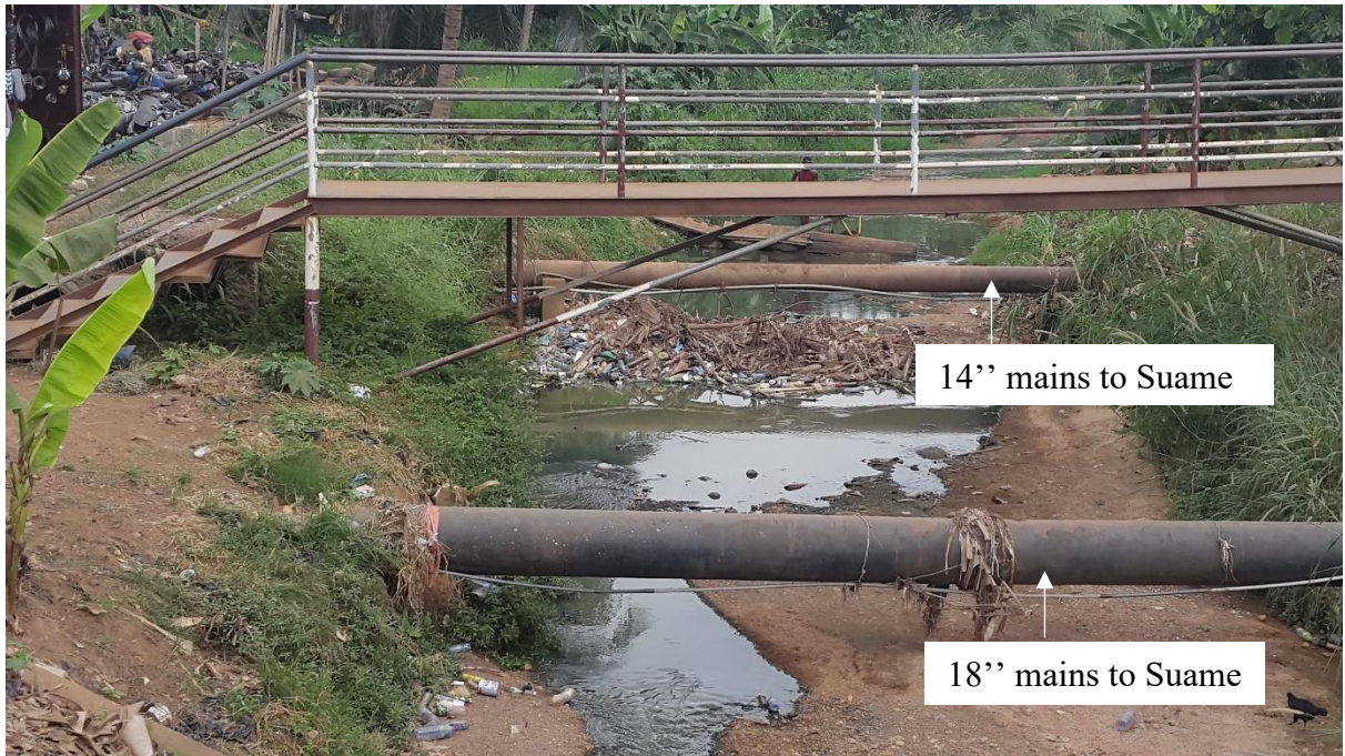
Figure 2.12 18-inch and 14-inch mains from OWTP to Suame Water Reservoir
