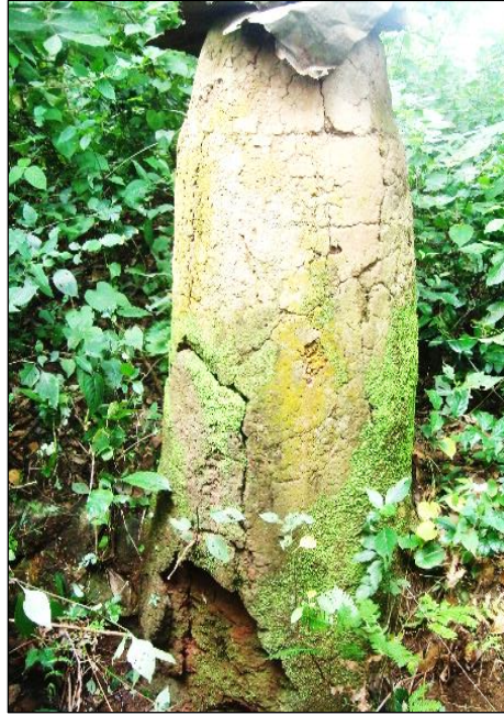
Figure 2.8 Photograph of Current State of Furnace
