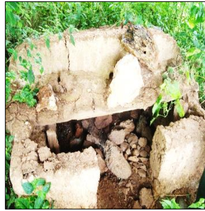
Figure 2.11 Destroyed Fire Trench
