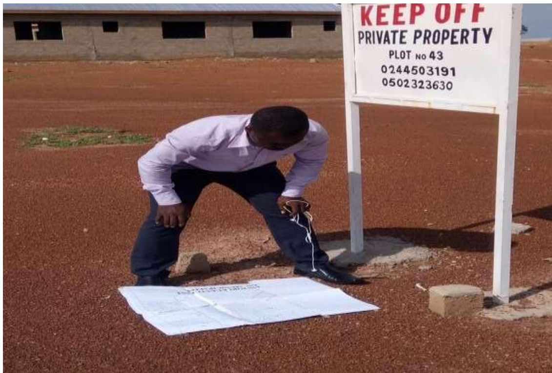
Fig 4.2 Site Reconnaissance to Relate the Layout to the Ground Pillars
