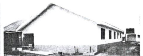
Rehabilitation of a community health post at Kpando in the Kpando District of the Volta Region. Project is over 95 per cent complete.
