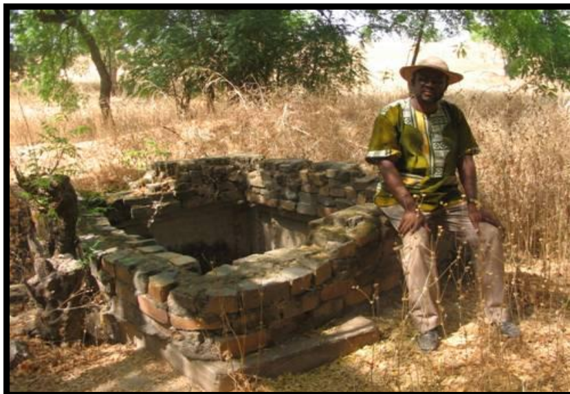
Fig. 2 The collar of the shaft at Nangodi which has been demolished recently by artisanal and small scale miners
