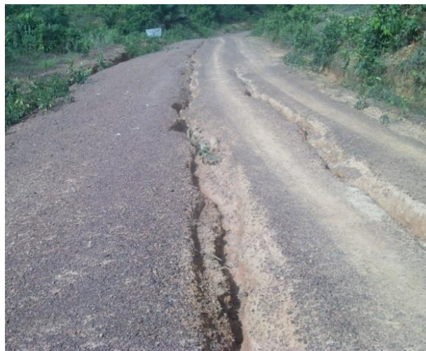
Fig. 1 Section of Road from Akwidaa to Cape Three Points
