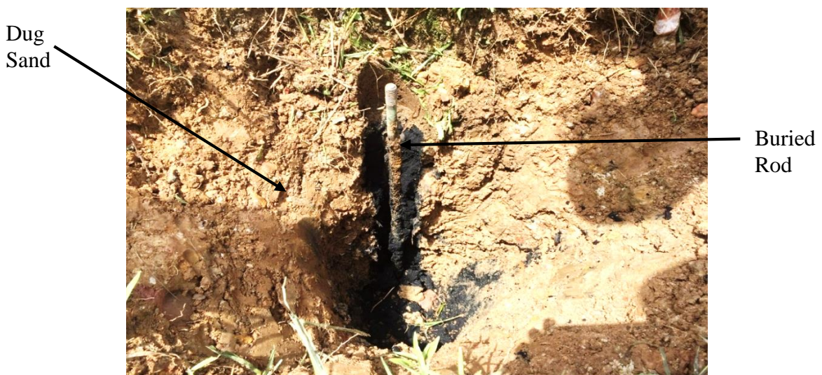
Figure 3.18 Rod Being Dug Out
