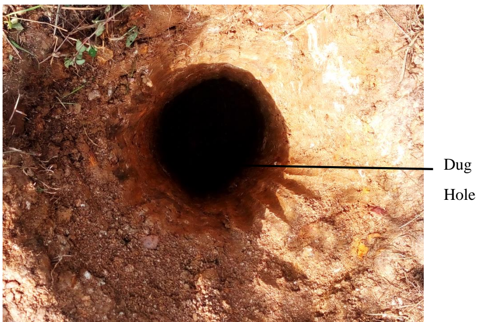
Figure 3.9 A Dug Hole for the Rod
