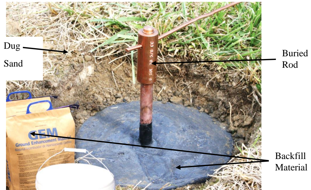
Figure 2.14 A Permanent Backfill Material Being Installed
