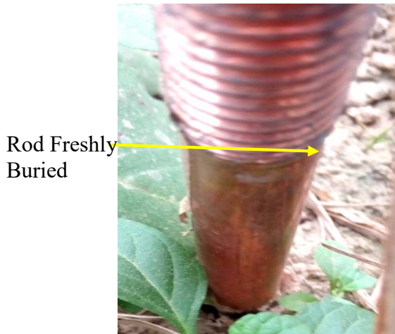
Figure 5.4 Freshly Buried Rod
